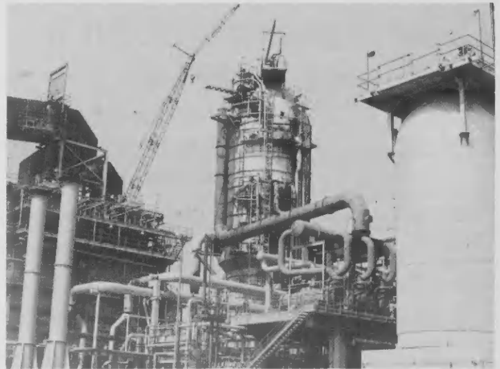
Two refinery units are undergoing major turnarounds. Above: the vacuum tower during the V3AR turnaround activities. Below: employees are inspecting the new pigtails at the H3AR unit.
